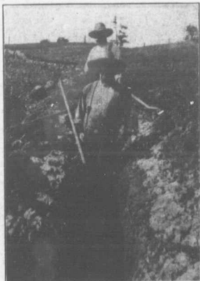
Under-draining on the farm of Mr. Geo. McKenzie, Thornhill, Ont. The illustration shows Mr. McKenzie in the background. The other man is Mr. John Simpkins of Thornhill, an expert in under-draining. See adjoining article.
