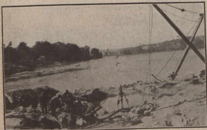
FIG. 11—EXCAVATION FOR TAILRACE AT GENERATING STATION SITE
