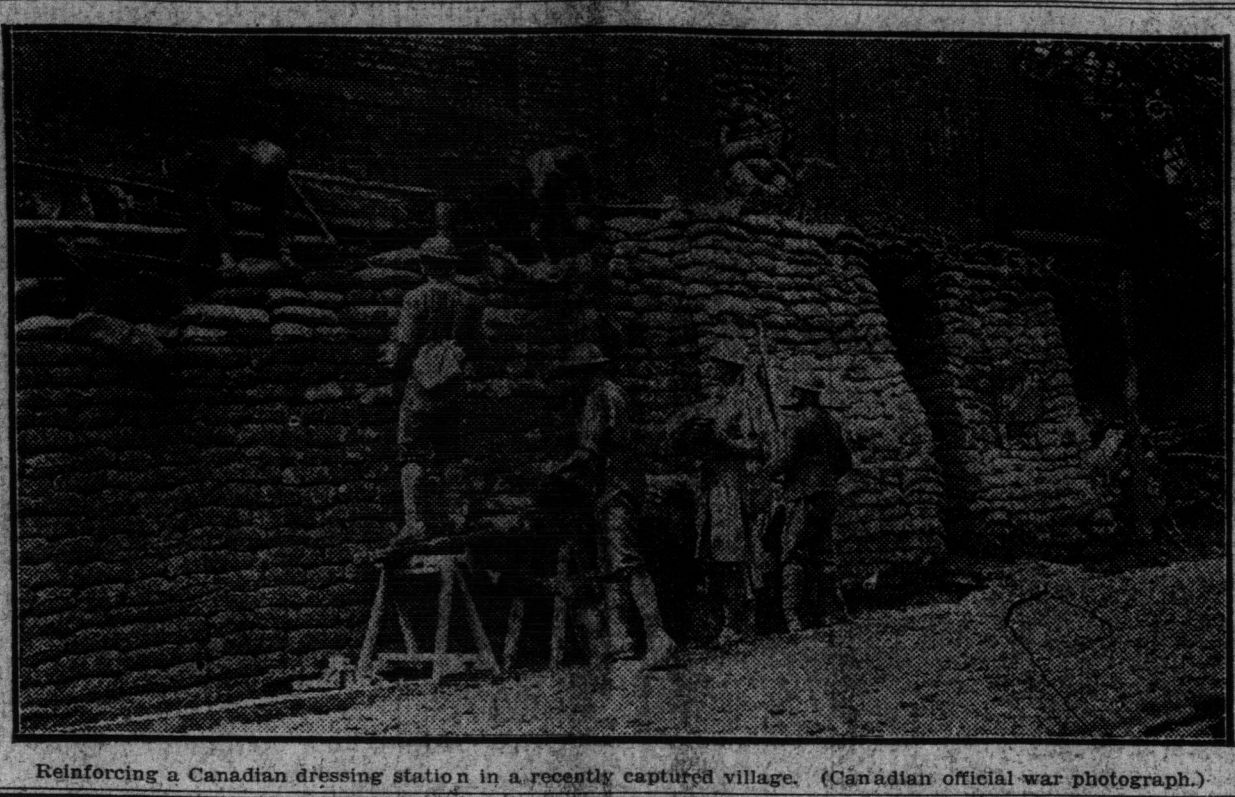
Reinforcing a Canadian dressing station in a recently captured village. (Canadian official war photograph.)
