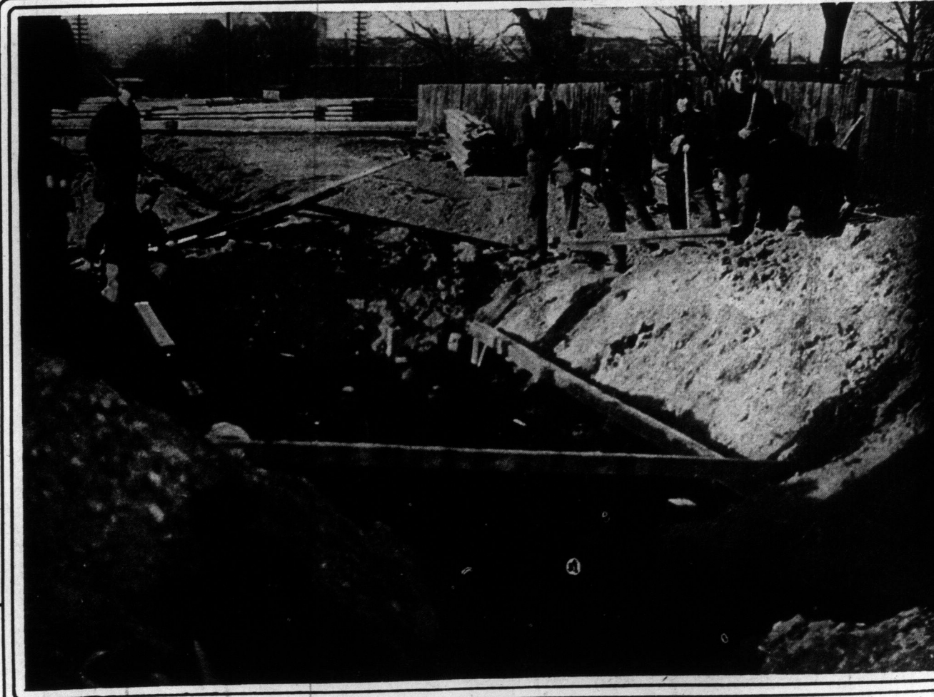
New kinks in trench warfare. Construction of a dressing-room for wounded at the Old Fort. It will be covered by seven feet of earth, and reached by trench tunnels when completed.
