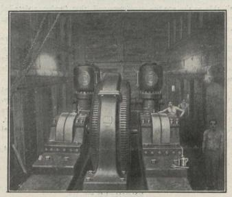
horse-power type "C" Westinghouse induction motor drove the 634 × 8-inch Knowles triplex pump at the uppermost pumping level.
