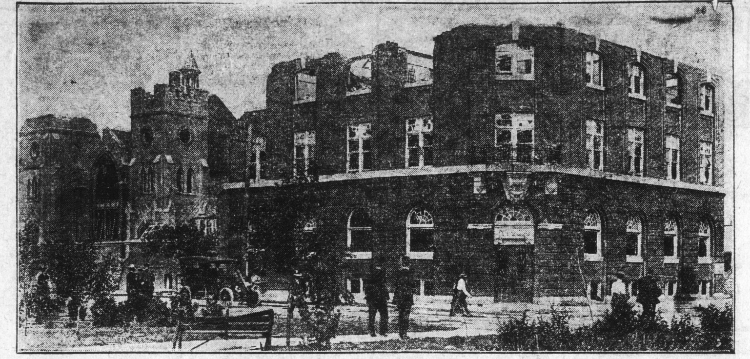
FINE BUILDINGS AT REGINA WRECKED BY CYCLONE—The structure on the right is the Knox Presbyterian Church, with the huge wind tower, the roof completely carried away, and the left tower shattered.
