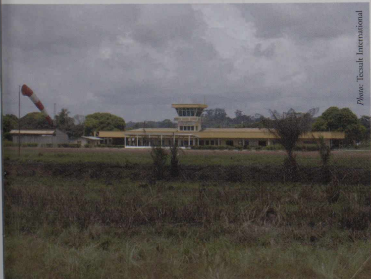
Tecsult International's provincial airports rehabilitation project, Lambasena Airport, Gabon
