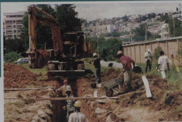
Tecsult International's wastewater system rehabilitation project, Antananarivo, Madagascar
