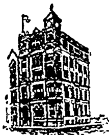
HEAD OFFICE BUILDING, MONTREAL.
