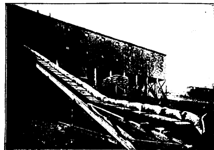
Freight and Package Elevator
