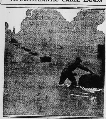
of them all, is landed at Far Rockaway, Long Island. The eastern terminus of the cable is Penzance, England. The cable line is indicated by the series of black casks seen in the photo, the man at the shore
