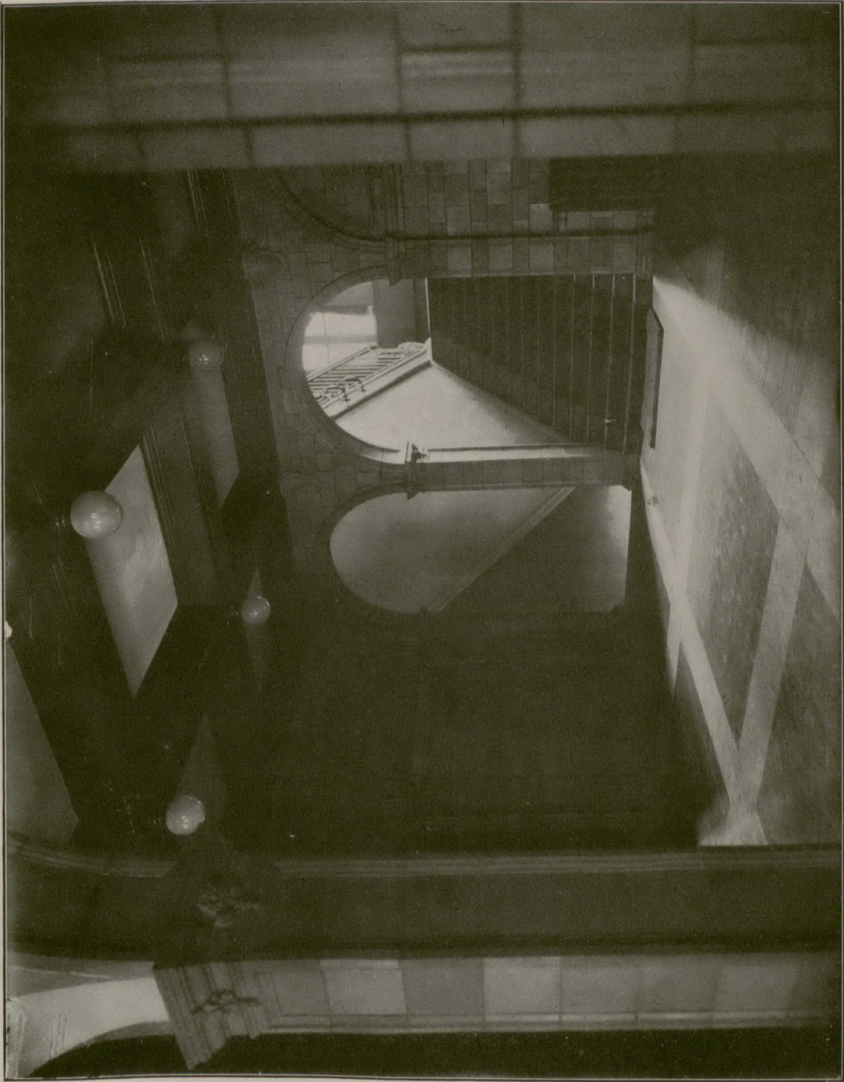
GROUND FLOOR HALL AND STAIRCASE.
