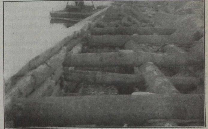
Detail of Crib Work, Page's Wharf
