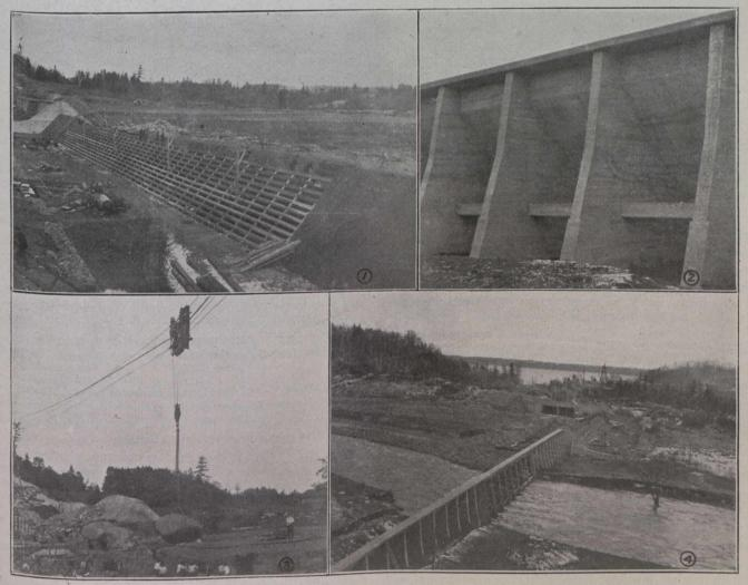
(1) View of Spillway from West Side. (2) Type of Abutment Construction, West Side. (3) Removing a 5-Ton Stone from Dam Site. (4) View of Dam, Spillway, Intake and New Course of Jacques Cartier River.
