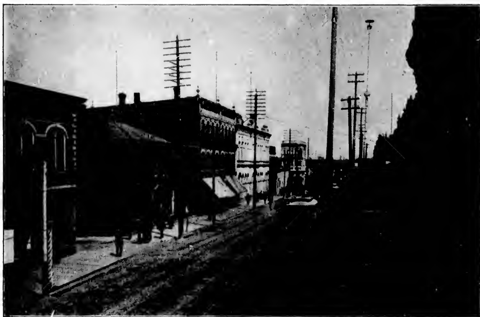
VIEW ON GOVERNMENT STREET, LOOKING NORTH.
