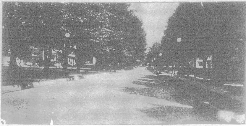
Brant Road, Galt, Ont. Constructed with "Tarvia-X," 1911, treated with "Tarvia-B," 1916.
