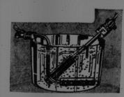
Just put water in cup or pitcher, drop in the heater and turn on the current. Hot water
