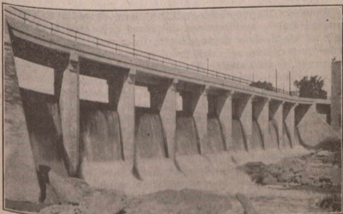
FIG. 2—A CLOSER VIEW OF THE DAM
