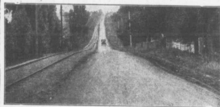
Kingston Road, Scarborough Township, York County Highway Board, Ontario. Treated with "Tarvia-B" in 1915 and 1916.
