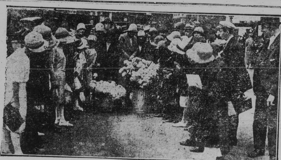
This photograph, taken in Trafalgar Square, London, shows the opening of the first canister of Canadian peonies, donated by Mr. W. Ormiston Roy of Montreal and shipped in cold storage.
