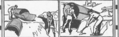
These pictures show how easily and quickly you can lay Pedlar Cultvert. Comes nesting, half-section within half-section—savings freight and cartage. Triple-lick flat flange locking ribs on each side are clamped together by a simple tool—no bolts nor rivets needed. The joints are lock-tight—only cultvert you can lay that will stand frost, and will stand tremendous strains. Won't leak, nor buckle, nor crack from frost. Cheaper than wooden culverts.
