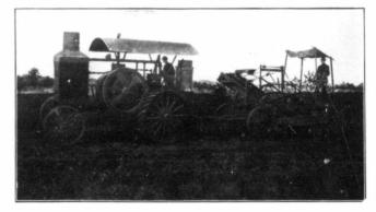
Hauls blade graders, elevating graders, drags, levelers and rollers, with the same sure, steady pull, even on turns. The finest kind of an outfit for pulling stumps and plowing when opening up entirely new roadways.
