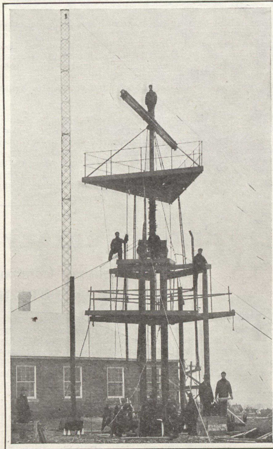
Beginning to Build the Big Steel Tower at Newcastle, Beside the Receiving Station. In the distance a 300-foot Wooden Tower Completed.
