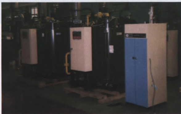
Available in capacities of up to 9 700 000 Btu/h, the Miura EX Series of boilers achieve full steam within five minutes.
