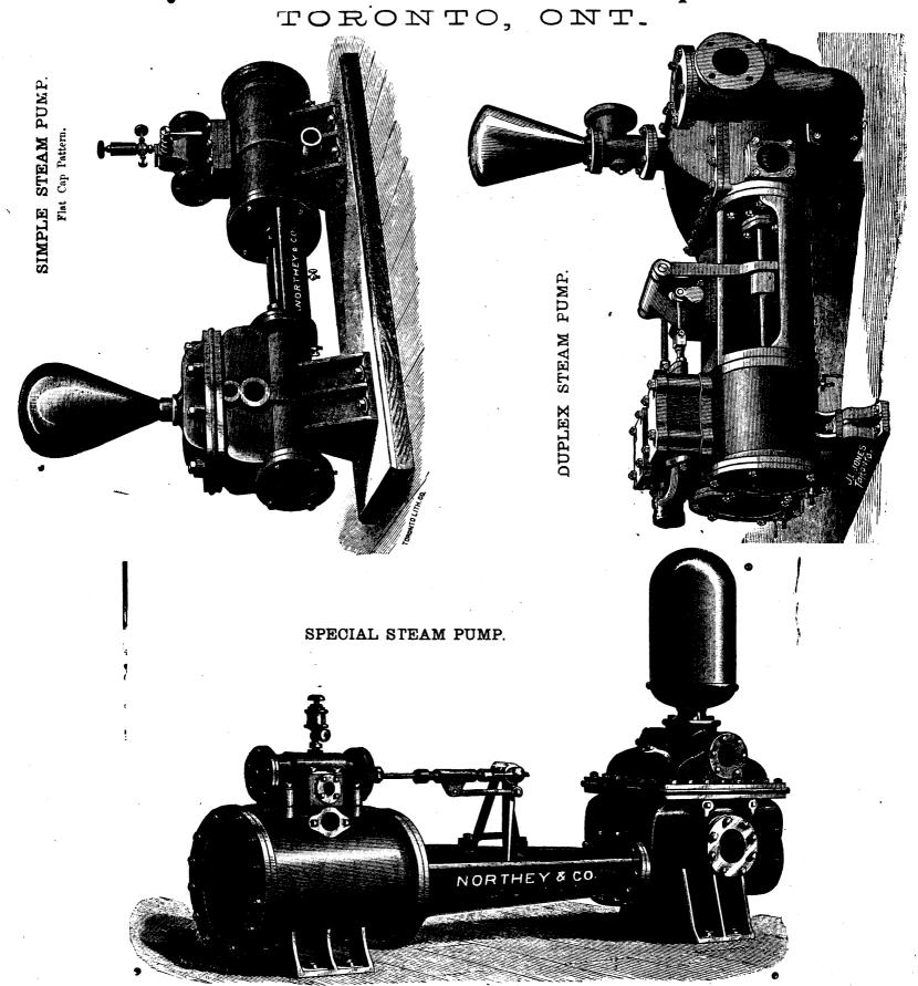
Steam Pumps of the best and latest designs for mining purposes, Boiler Feeding, Fire Protectio, and General Water Supply, etc.
