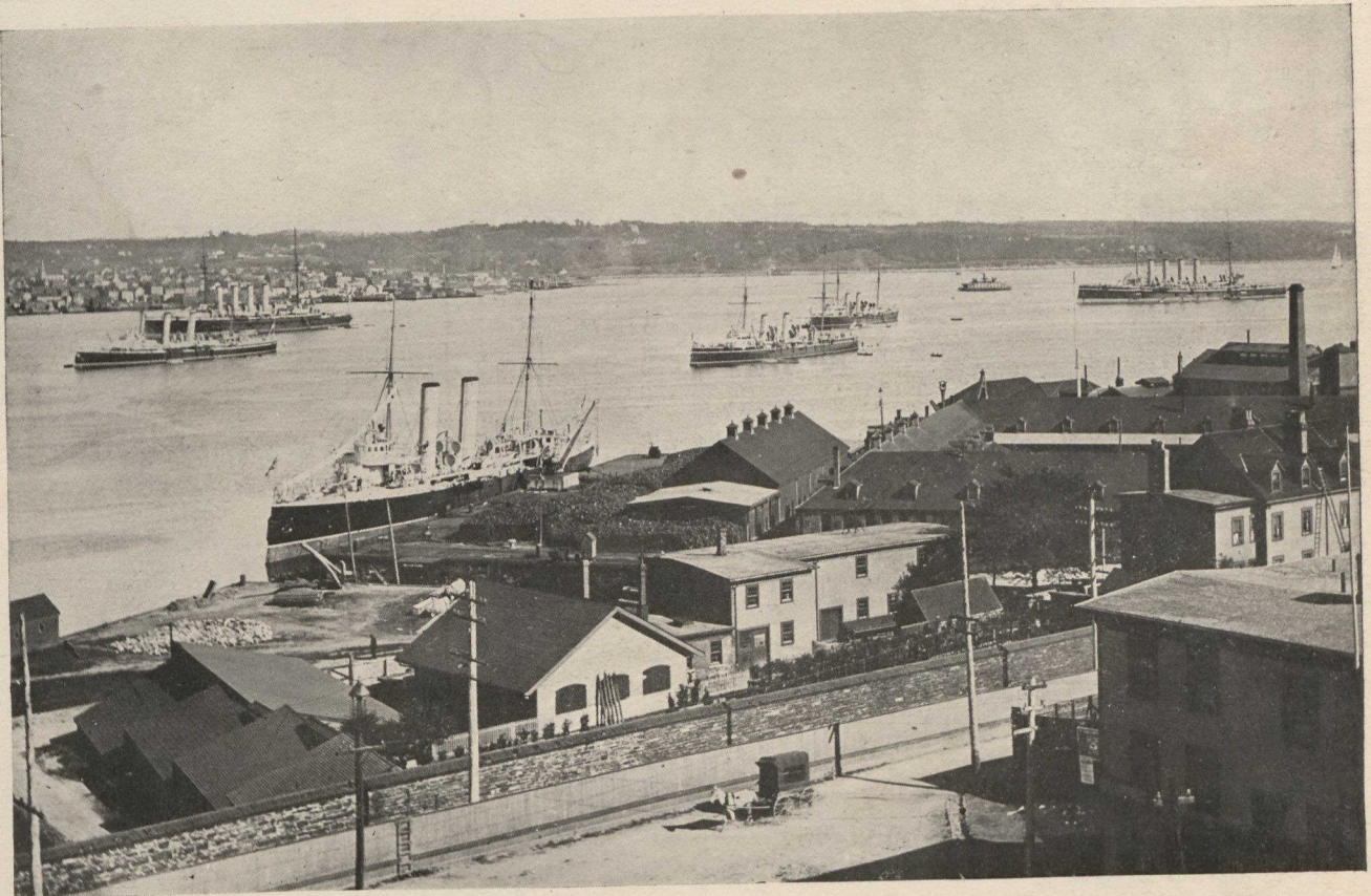
HALIFAX DOCKYARD, TAKEN OVER BY CANADA JANUARY 1st.
