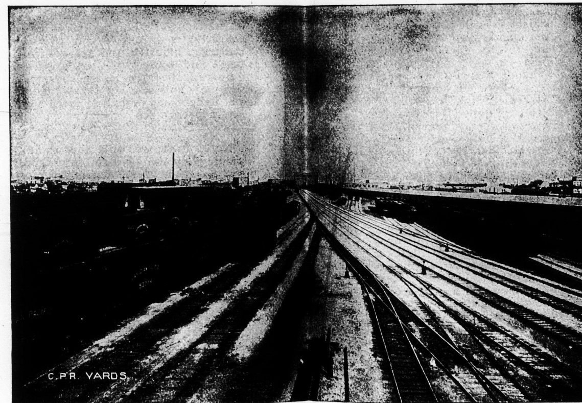
C.P.R. Yards—Looking East from Overhead Bridge.
