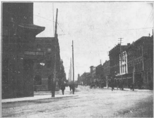
Second Ave. Looking South
