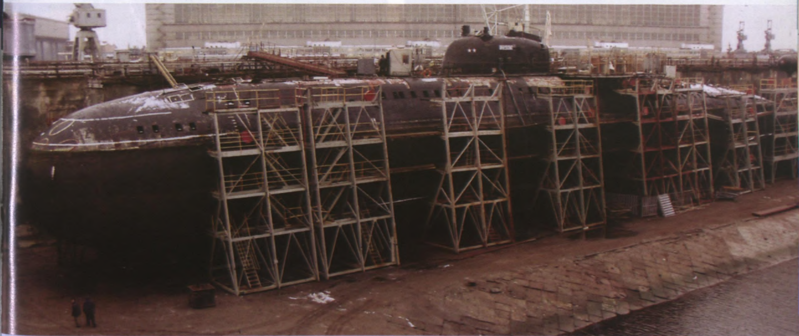
Victor III being dismantled in dry dock
