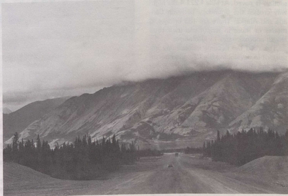
Alaska Highway near Haines road junction in the Yukon.
