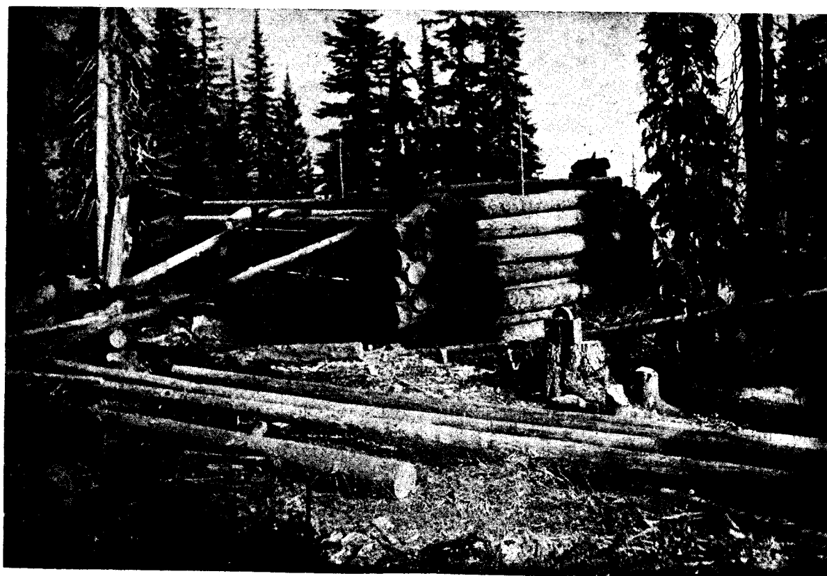
Empire Cabin under construction, Aug. '99.
