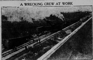
St. Catharines, Ont., completely blocking east and west lines. The huge cars were flung right and left off the tracks. The picture shows a wrecking train at work with its powerful derricks, removing the wreckage from the
