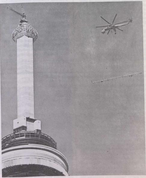
The Skycrane helicopter at work, settling one of the 39 steel transmissionmast sections in place on Toronto's CN Tower - soon to become the world's tallest free-standing structure. It is estimated that it will take 30 working days to complete the task of erecting the 335-foot mast, and early this spring, the CN Tower will reach a height in excess of 1,800 feet.
