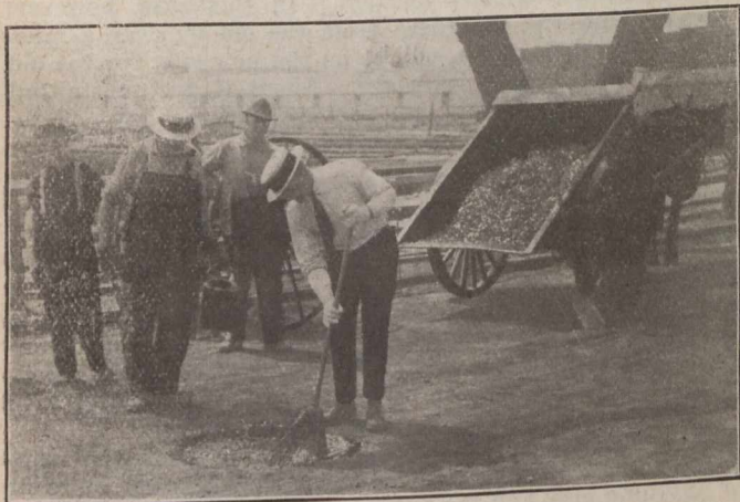
FIG. 4—PAINTING BOTTOM AND SIDES OF HOLE
