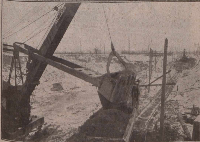
FOUR VIEWS OF ONE OF THE 8-YD. SHOVELS WORKING IN EARTH—TOP LEFT PHOTO SHOWS SOME RIP RAP IN PLACE—TOP RIGHT, TRAIN BEING LOADED AT STA. 346+81—BOTTOM LEFT, WORKING SOUTH OF THE WABASH R'Y—BOTTOM RIGHT, WORKING AGAINST A HIGH FACE AT STA. 346+81
