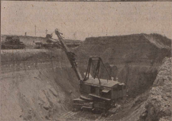
FOUR VIEWS OF ONE OF THE 8-YD. SHOVELS WORKING IN EARTH—TOP LEFT PHOTO SHOWS SOME RIP RAP IN PLACE—TOP RIGHT, TRAIN BEING LOADED AT STA. 346+81—BOTTOM LEFT, WORKING SOUTH OF THE WABASH R'Y—BOTTOM RIGHT, WORKING AGAINST A HIGH FACE AT STA. 346+81
