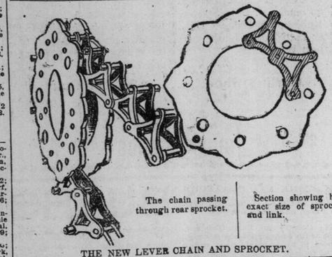
Section showing half through rear sprocket, exact size of sprocket and link.
