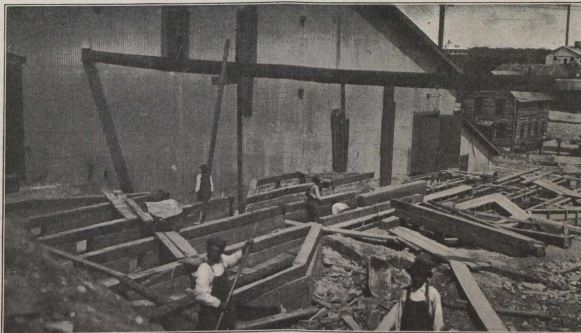
Constructing Foundations for Addition to McIntyre Plant
