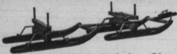
The U.G.G. Sleighs have selected hardwood in all wooden parts. The runners are of straight-grained oak, BENT TO FORM—not sawn. All parts where strain or wear comes are protected with steel bands. There are steel straps running 18 inches back from the nose of each runner. The draw rods passing through these straps put the strain of draft on the body of runner instead of the nose, as is the case in many sleighs
