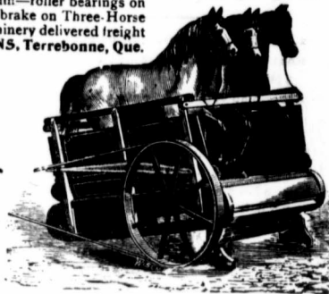
THREE-HORSE TREAD POWER with roller bearings
