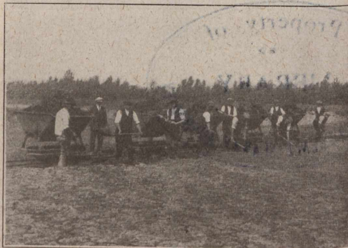
FIG. 8—FILLING WAGONS WITH DRY SLUDGE
