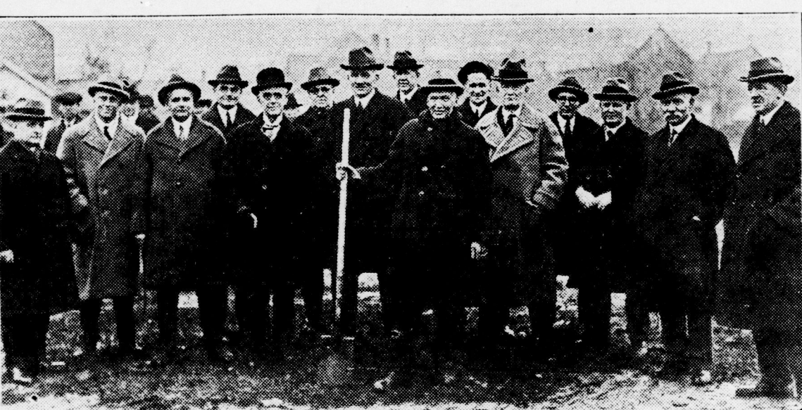
FIRST SOD TURNED FOR NEW ST. THOMAS SCHOOL.
