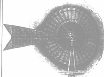
The wheel is built on a hub revolved on a long stationary steel spindle. As a result there is less friction.
