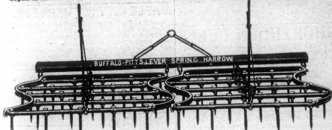
Spike Tooth.—Supplied in two or three sections of 50 or 75 teeth as desired, with freeing from rubbish. Safety relieving spring to prevent jumping or injury from fixed obstacles.
