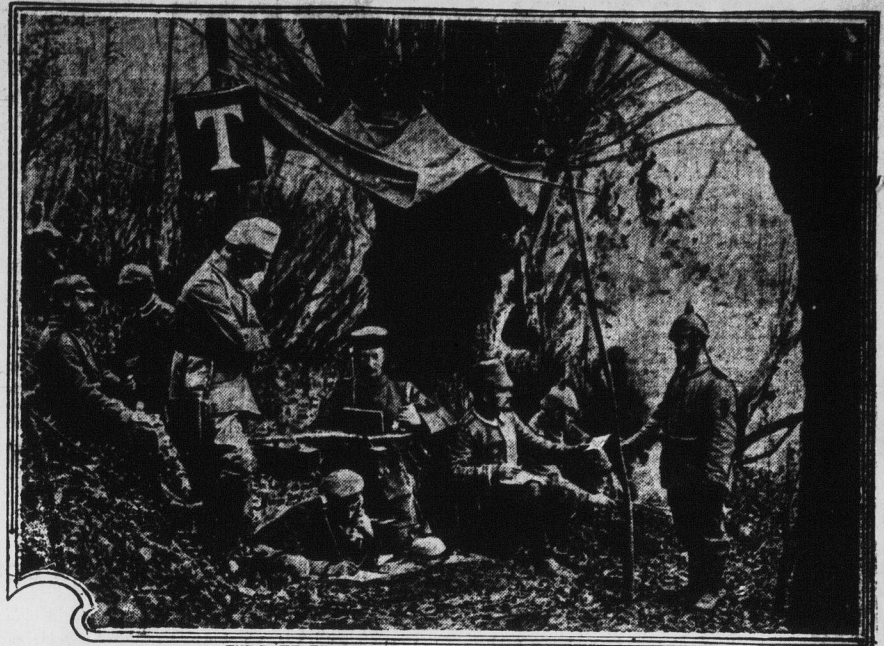
Field telephone station on the banks of the Aisne. The instruments are carried by the different regiments, and when camp is made they are put up and made ready for use. These stations are situated all along the lines and messages are given and received by the operators.
