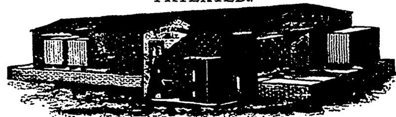
COST of erecting, running and maintaining the lowest and results the highest of any dry kiln and drying system in the market. Green Elm, Ash, Whitewood, &c., for furniture dried in six days; only exhaust steam 10 hours per day used.
