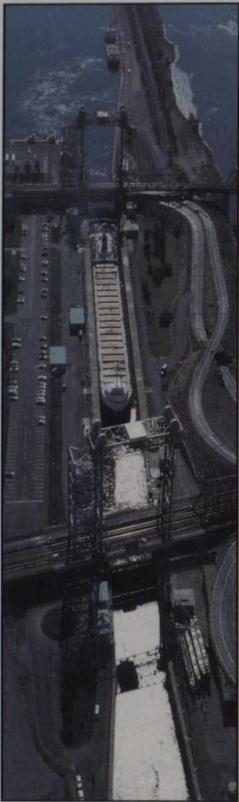
A laker, — a cargo ship specially designed for the Saint Lawrence Seaway, — passing through the Saint Lambert lock
