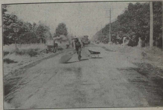
Fig. No. 6.—Sanding Over the Squeegee Coat
