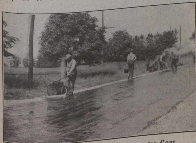
Fig. No. 5.—Putting on the Squeegee Coat
