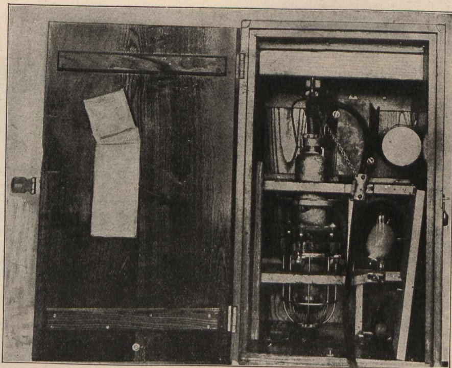
Fig. 2.—Submarine Electric Lamp and Accessories: Packed for Transport.
