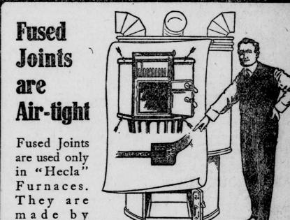
of the radiating chamber to a white heat and fusing the metals into one piece-making a joint so permanent and so tight, that it prevents for all time the escape of smoke, gas and dust into the house.
