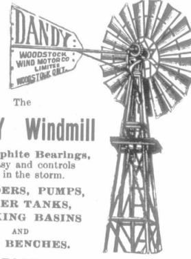
with Graphite Bearings, runs easy and controls itself in the storm.
