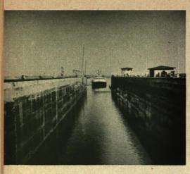
Left: Côte Ste. Catherine Lock has a lift of 30 feet and requires 24,000,000 gallons of water to fill
